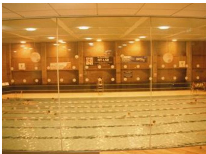
Image of main pool hall prior to the lighting and ceiling renewal
